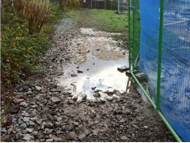
Silty material partially blocking French drain / Silty material partially blocking French drain
