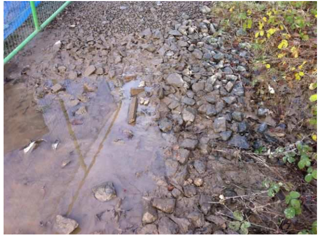
Silty material partially blocking French drain / Silty material partially blocking French drain
