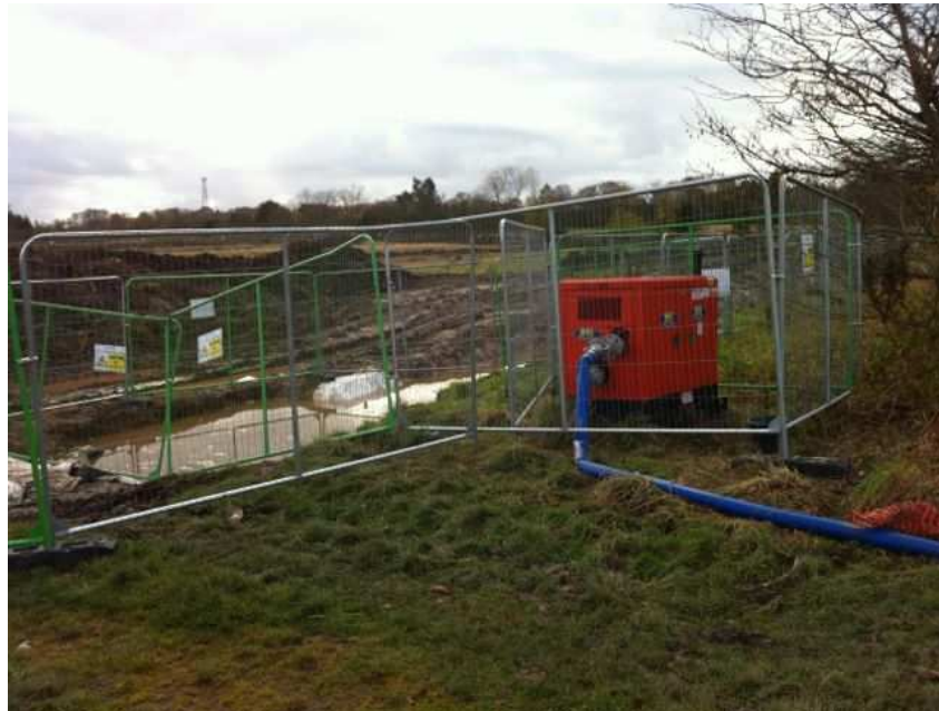
Water being pumped towards Hazledene Road to reduce water flowing Down towards sales pod site
