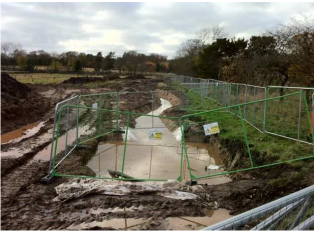
Towards top of Zone H, V-shaped trench to collect water / Water entering French drain
