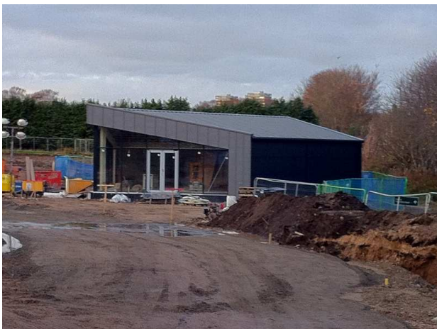
Drainage on Site
