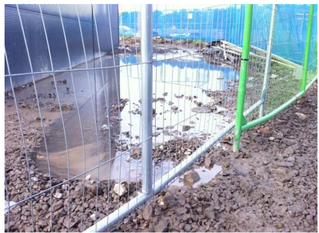
Towards top of Zone H, V-shaped trench to collect water / Water entering French drain
