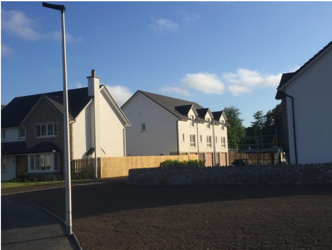
Houses nearing completion in Zone C including town houses
