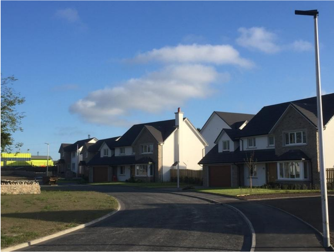
Houses nearing completion in Zone C
