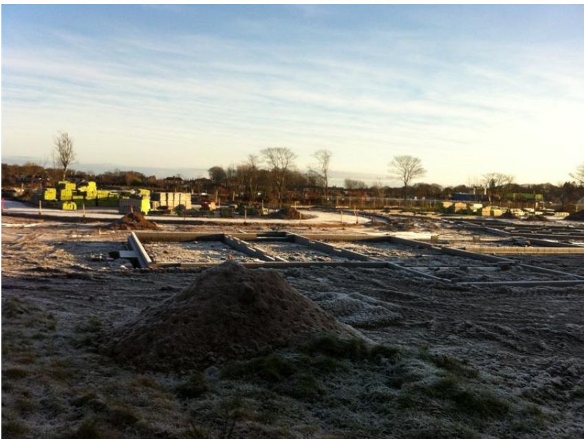
Foundations being laid in Zone A
