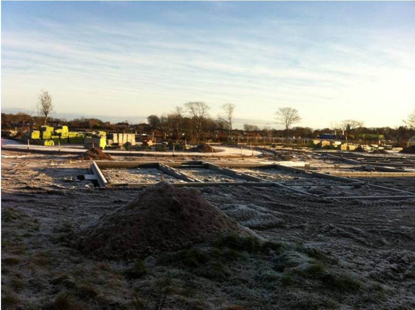
Foundations being laid in Zone A
