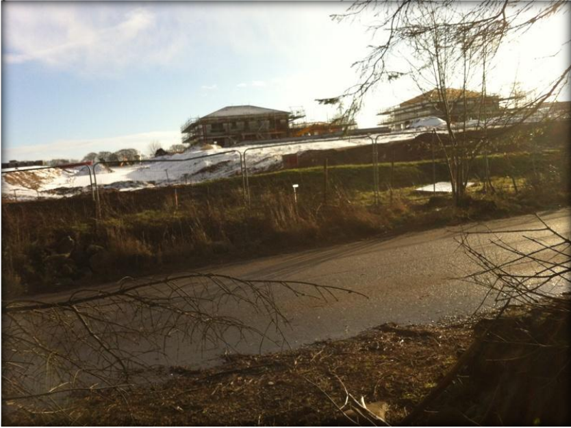
First Houses in Zone A, with access off Hazledene Road
