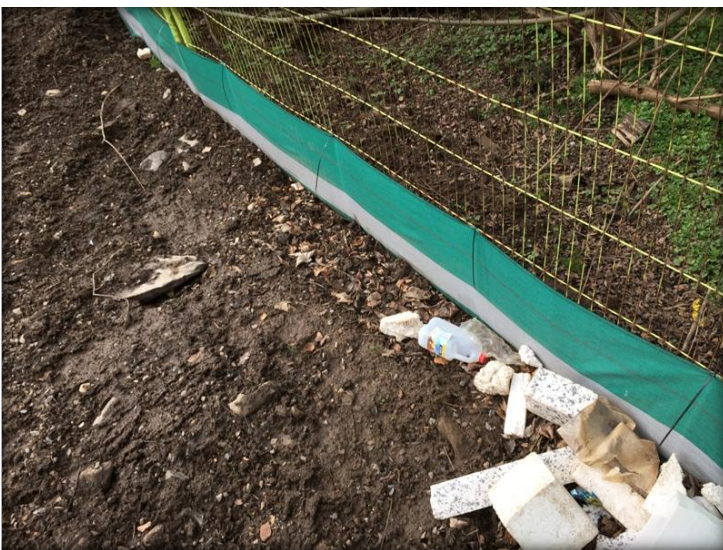
Milk container and polystyrene near north retention pond
