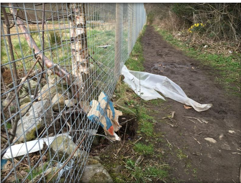
Core path with polythene blowing under fence
