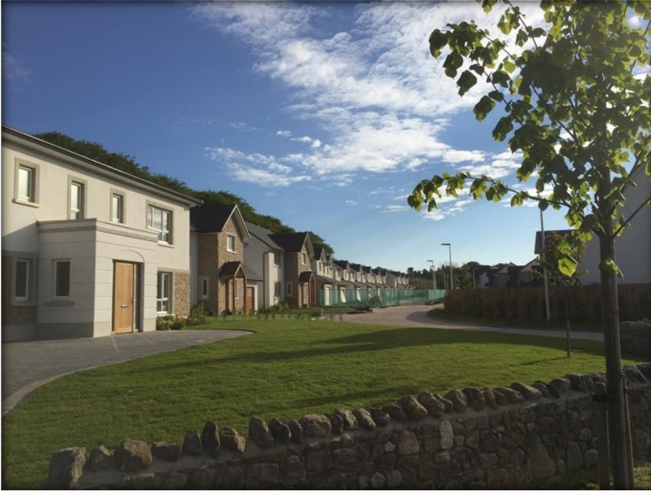
Houses in Zone H are nearly complete with more new residents moving in.
