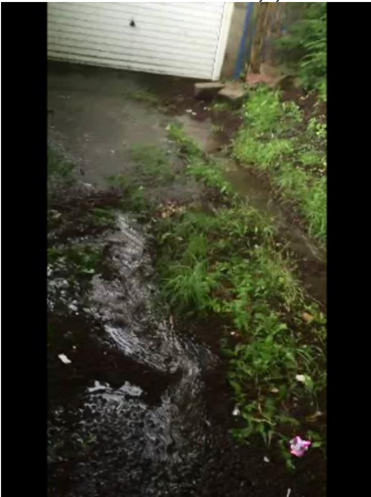
Flooding in the rear garden at NO.21 Pinewood Road
