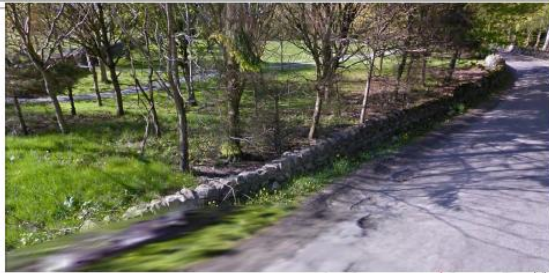
view of wall to be retained to north west side of road
