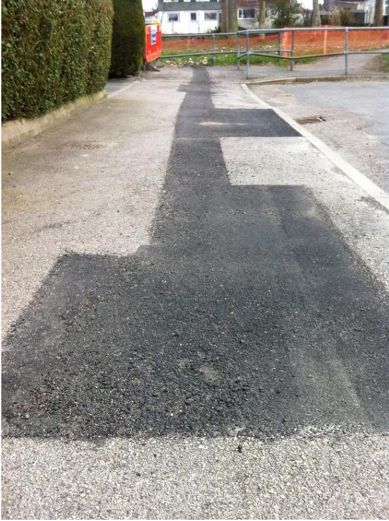
Initial Repair Dec 2013
