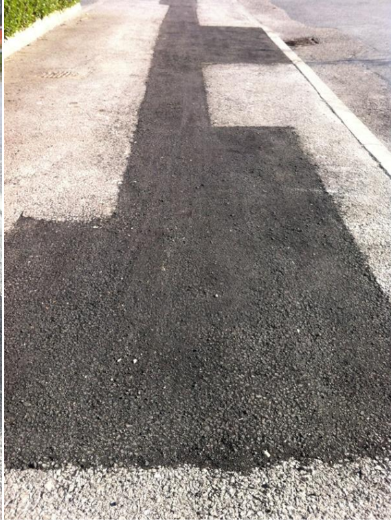
Second Repair in April 2014
