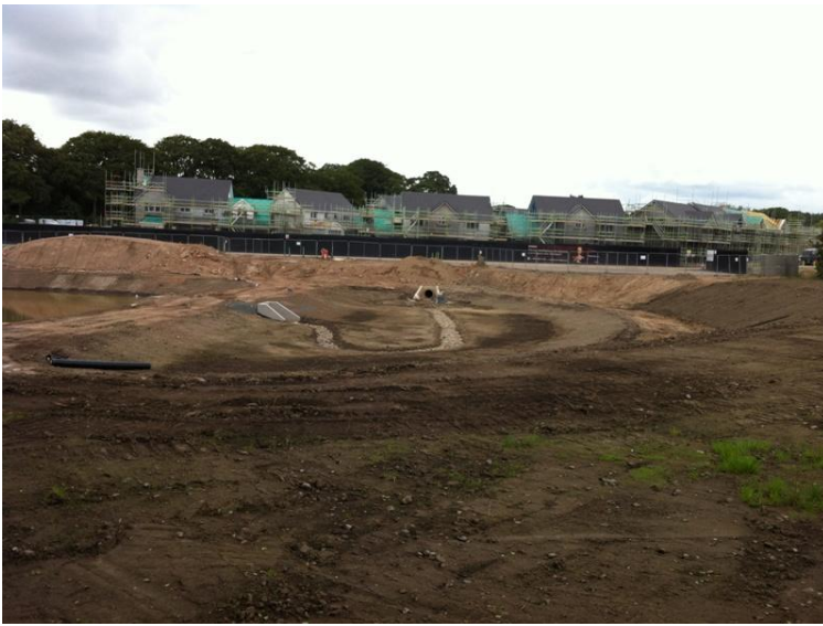
Top Retention Pond
