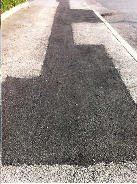
Second Repair in April 2014
