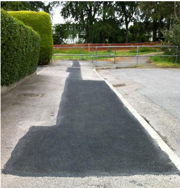
Third and Final Repair in May 2014
