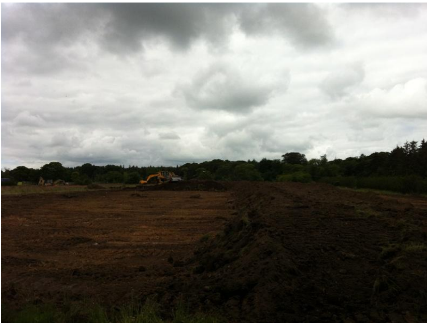
Land in Zone A being cleared – 27 th June 2014
