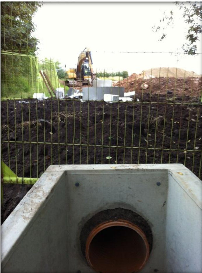
Outlet pipe connected to headwall
