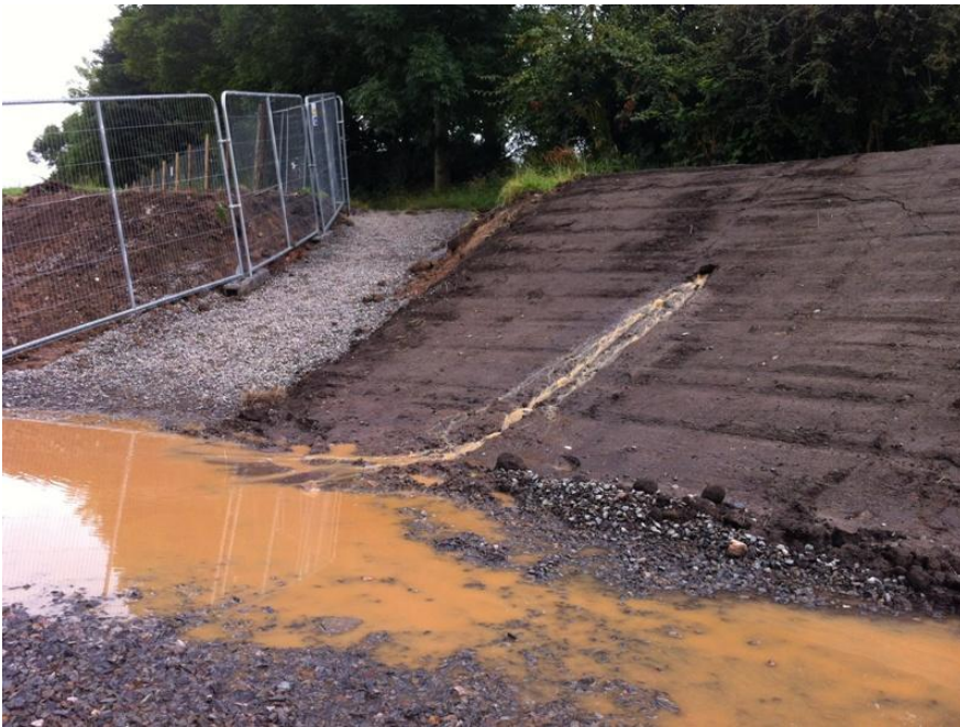
After heavy overnight rain, covered up field drain breaks through bank of soil flooding temporary path.
