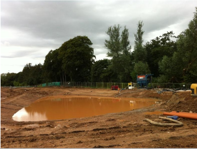
North Retention Pond in Zone A
