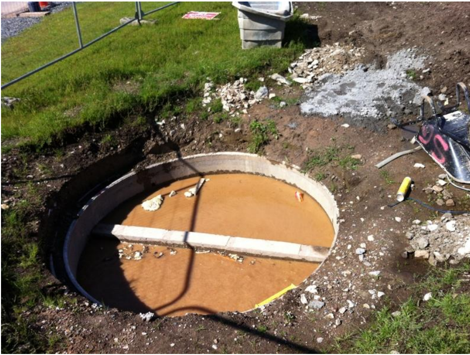
Hydro Brake manhole completely full
