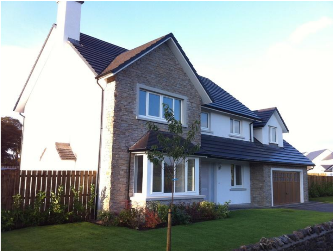
Zone H houses nearing completion ready to be occupied possibly in December.
