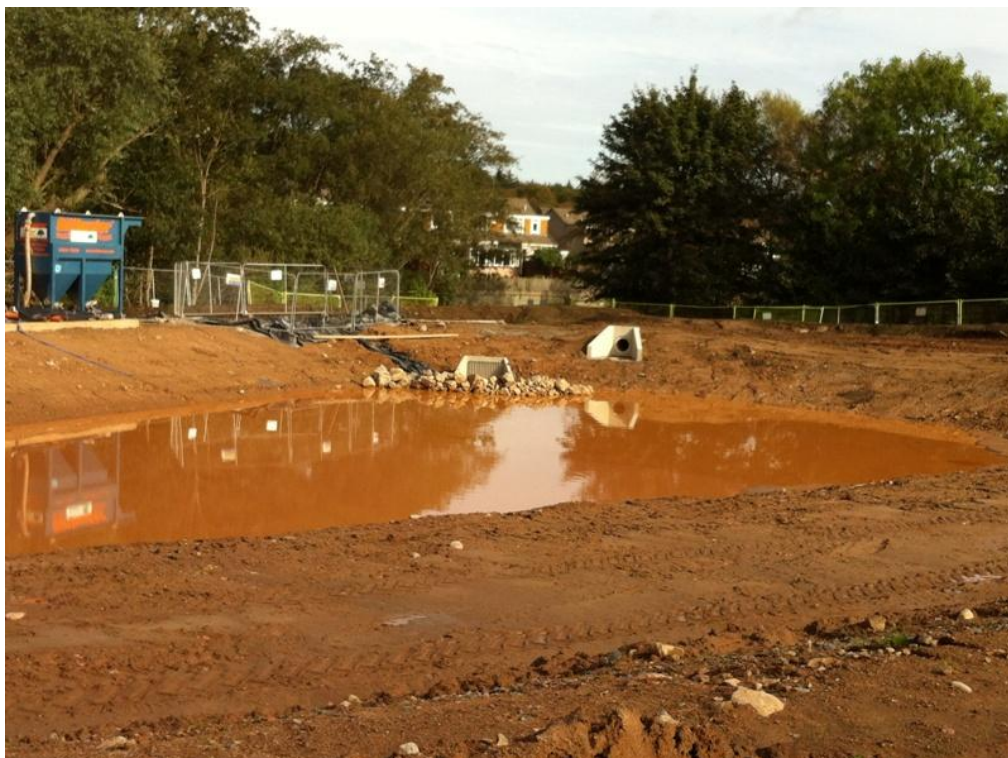
North Retention Pond
