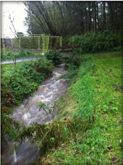
Burn downstream of north retention pond flowing very fast
