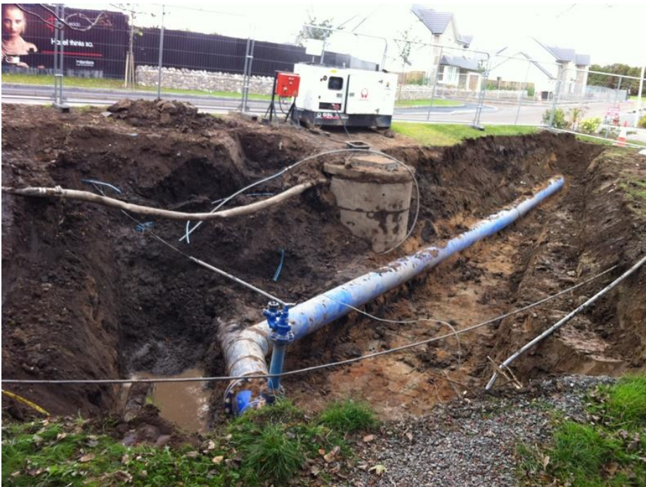
Work starts on diverting the main water main
