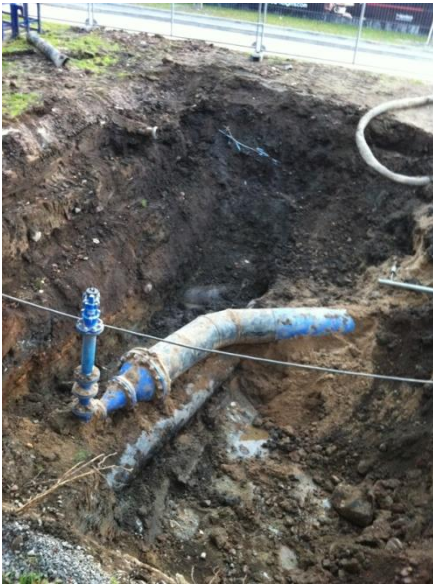
Work starts on diverting the main water main
