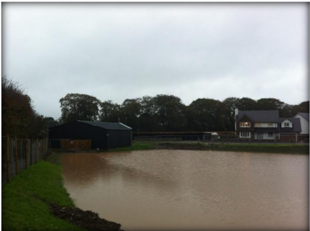
South retention pond very full
