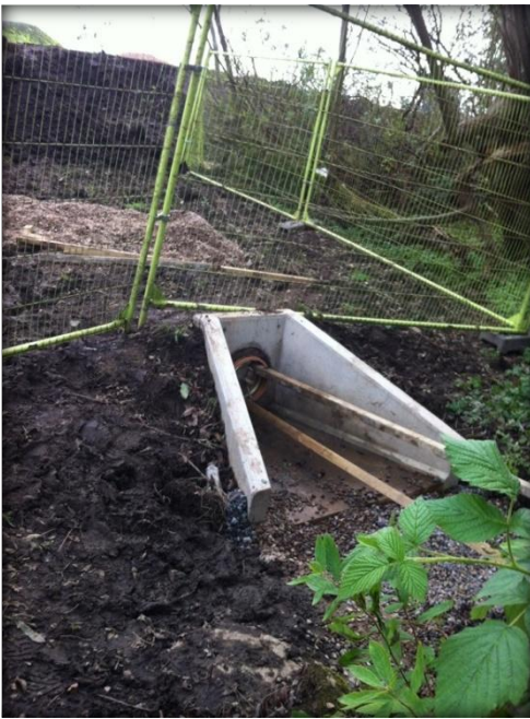
Attempt to seal outflow from north retention pond
