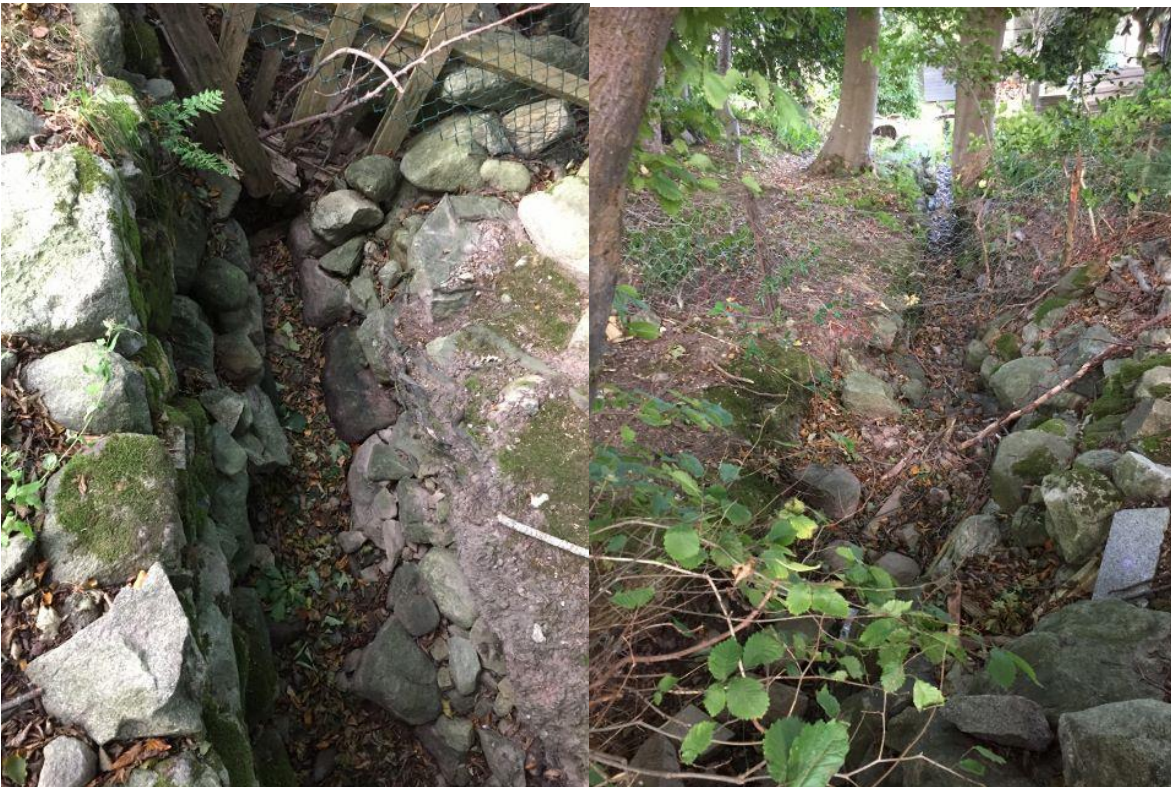
Un-named burn that feeds into Cooper's pond is now completely dry
