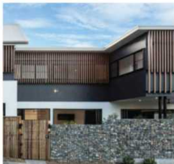
TIMBER EFFECT ALUMINIUM BATONS TO CLADDING AND WINDOW SURROUNDS
