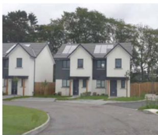
4 Ash3 House Type to the north in Zone F
