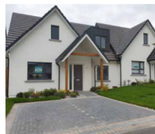
3 Rowan House Type to the north in Zone F
