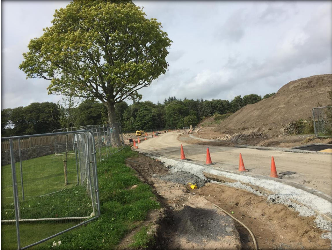
Dandara Hazledene/Pinewood Zone B work starts
